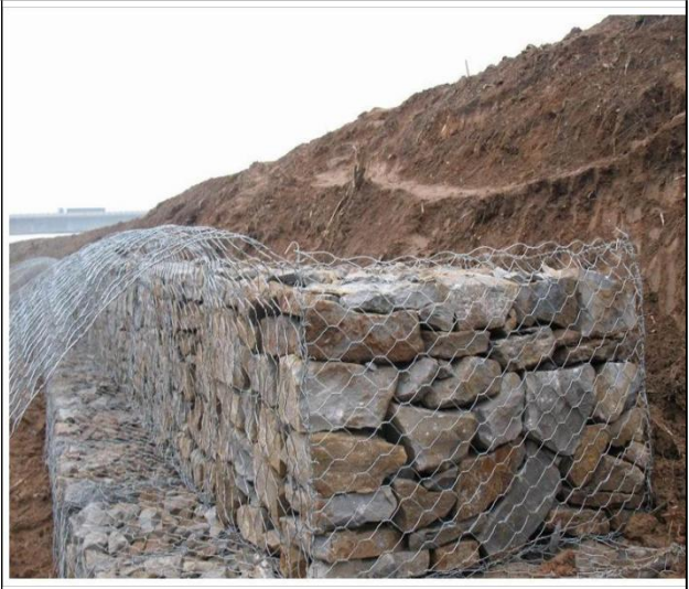
排土场区石笼挡墙
