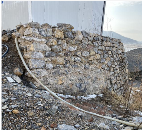
料场区浆砌石挡墙
