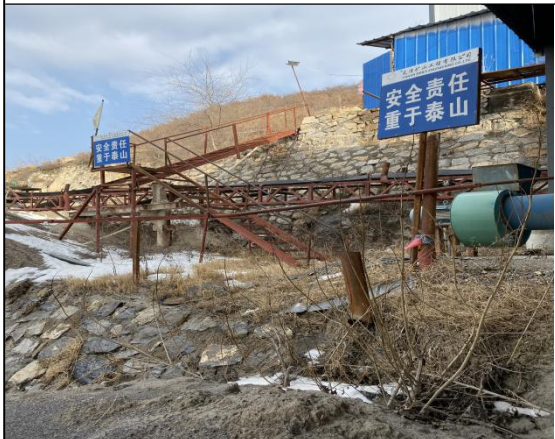
料场区浆砌石挡墙
