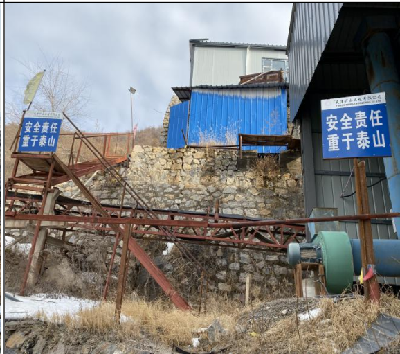
料场区浆砌石挡墙
