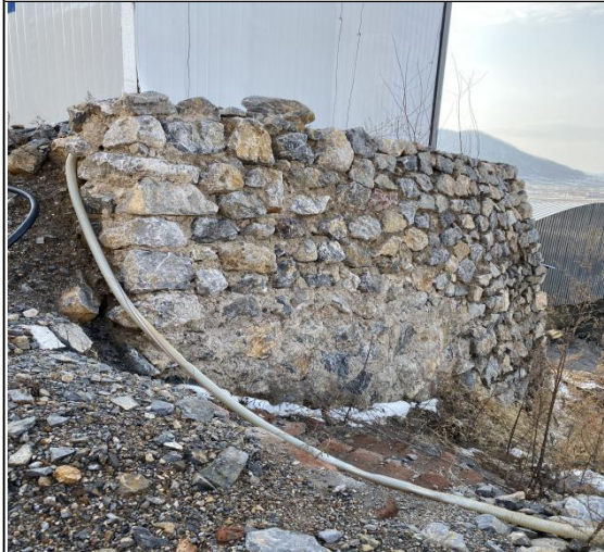
料场区浆砌石挡墙
