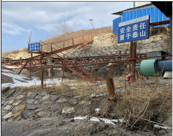
料场区浆砌石挡墙
