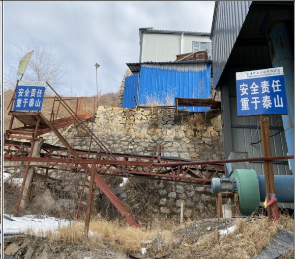
料场区浆砌石挡墙
